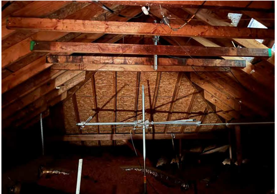
The author's attic antennas. His three-element, 6-meter beam is in the middle. If you look closely, you can see his two 20-meter dipoles and 6-meter loop.
