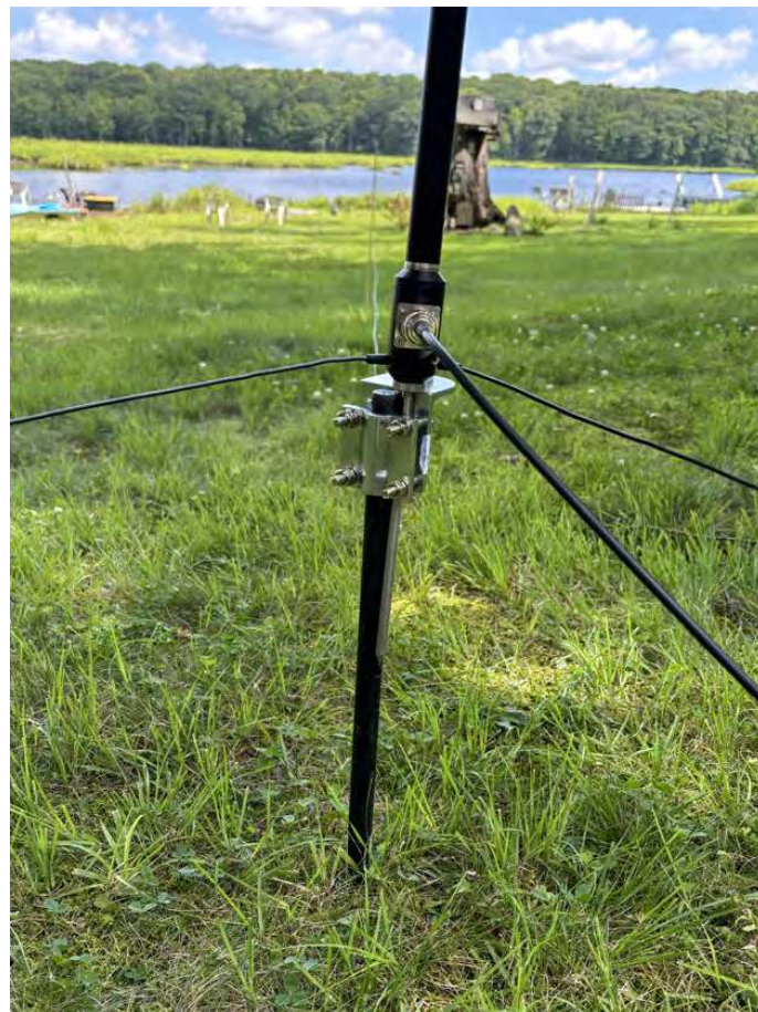
Figure 17 — The Radioddity HF-009 slightly elevated installation using a Home Depot metal stake and an available mobile bracket.
